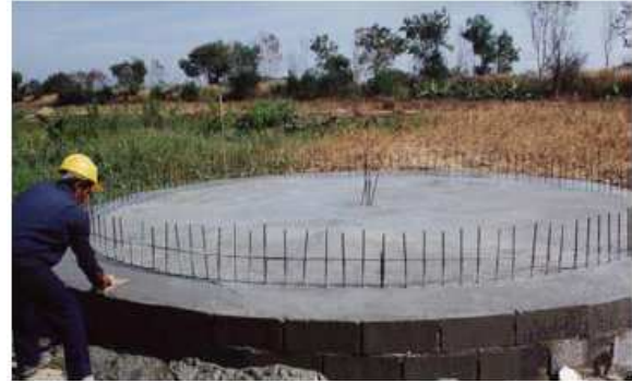
Figure 7. Casting of Concrete Base Slab
