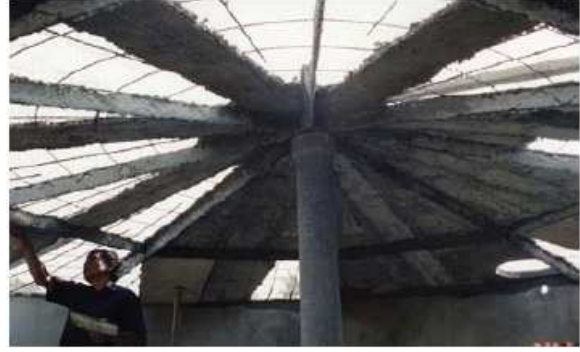
Figure 19. Plastering of Roof
