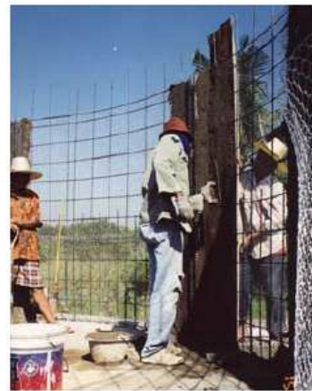
Figure 14. Plastering of Wall
