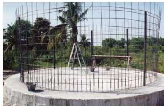
Figure 8. Vertical Reinforcement and Wall Stiffeners
