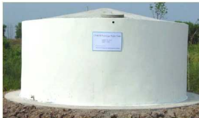
Figure 21. Finished Ferro Cement Tank
