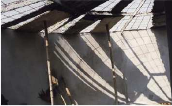
Figure 18. Temporary Formwork for Roof
