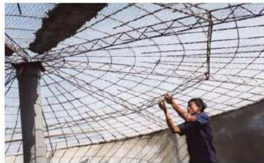
Figure 16. Placement of Roof Reinforcements
