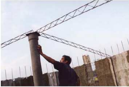
Figure 15. Fixing of Roof Trusses (Stiffeners)
