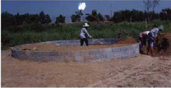
Figure 4. Preparation of Foundation
