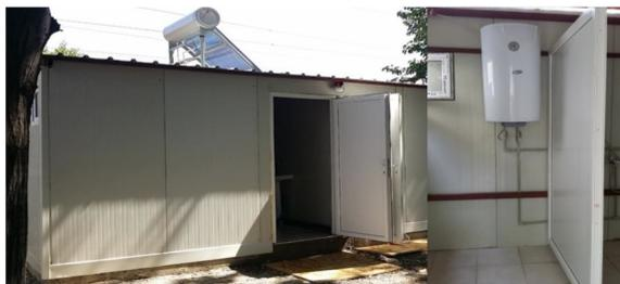
Pictures showing solar and boiler heating systems for showers.
