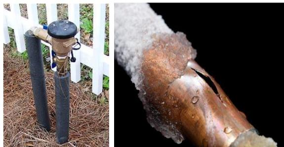
Picture showing insulation of water supply pipes outdoor and the damage freeze could cause to un-insulated pipes.
